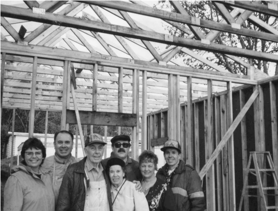
Our family building Leon & Liz's garage
